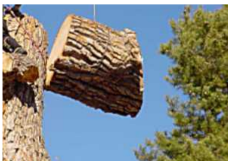
Affordable Tree Removal Services in Sarasota (Check out the Prices)
